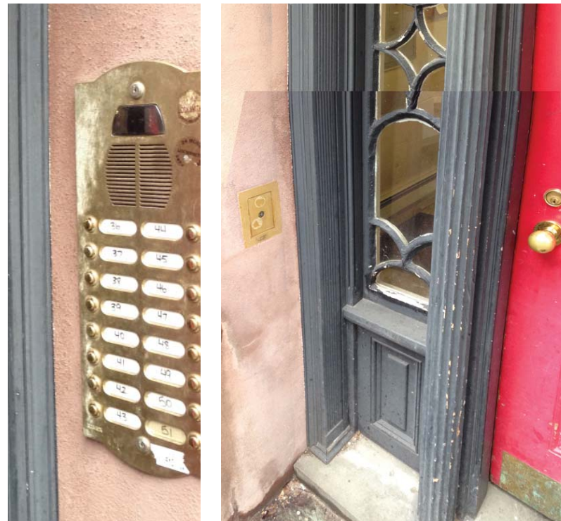
CLOSE UP OF EXISTING INTERCOM AND KEY BOX
