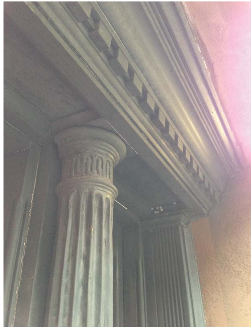
EXISTING DOOR SURROUND
