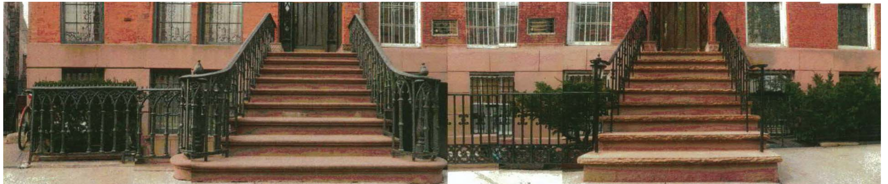
NEIGHBORHOOD PROPERTIES THAT ALSO SHOW STUCCO RUSTIFICATIONS
