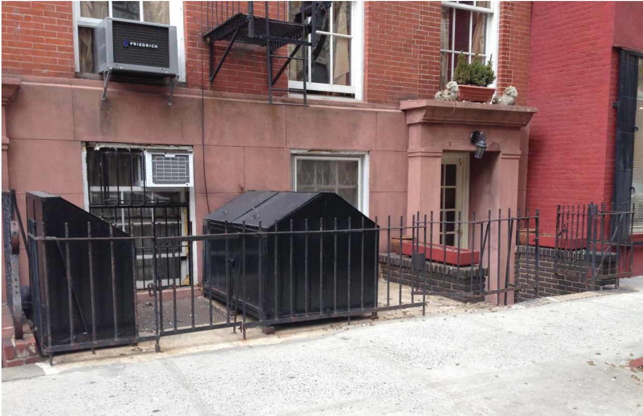
EXISTING FENCE ACROSS THE STREET AT 7 CHARLES ST.
