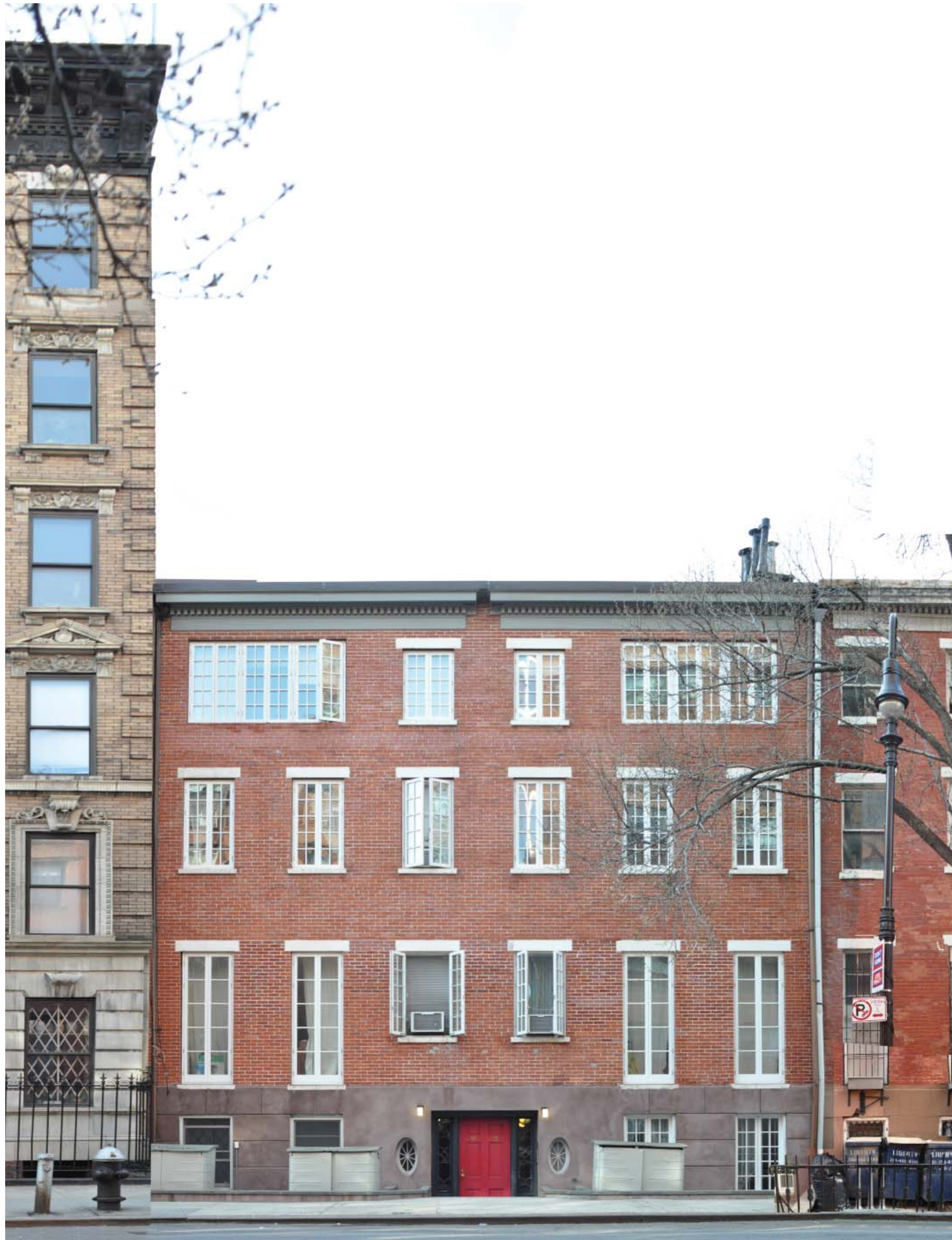
16-18 CHARLES ST., EXISTING FRONT FACADE
