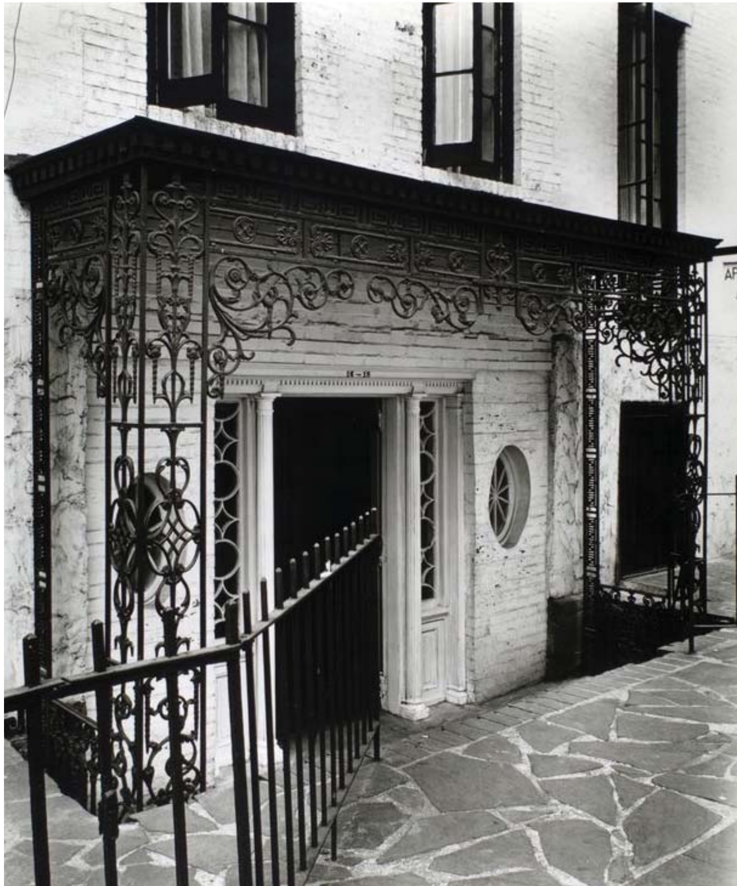
DOORWAY, 16-18 CHARLES ST., JUNE 01, 1938
