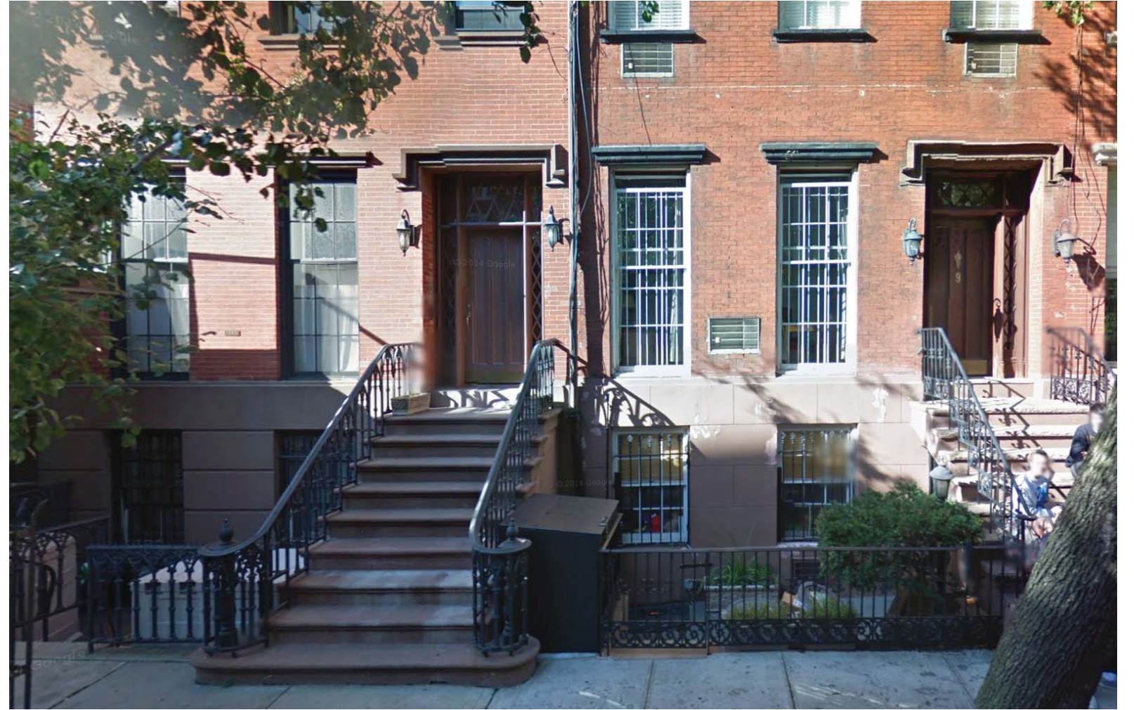
EXISTING STUCCO RUSTIFICATIONS AT 19 CHARLES ST.
