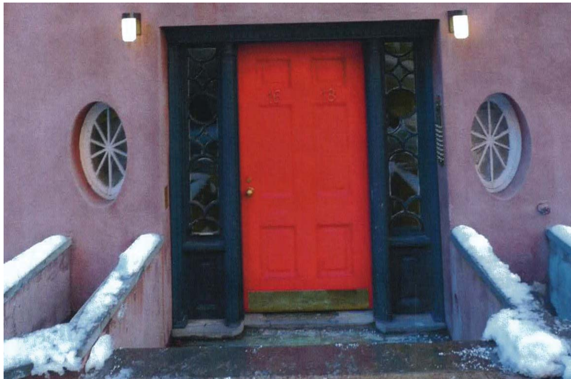
CURRENT RECESSED MOUNTED INTERCOMES ARE NOT OBTRUSIVE
