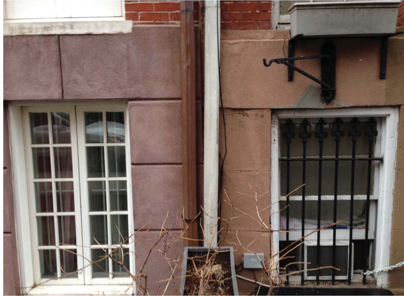
EXISTING STUCCO RUSTIFICATIONS AT 18 CHARLES ST / 20 CHARLES ST.
