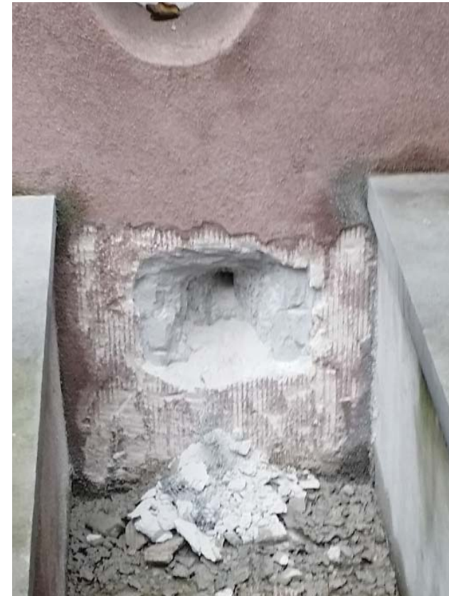
PROBE AT EAST SIDE OF ENTRY
